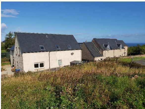
View north towards units 3 + 4
